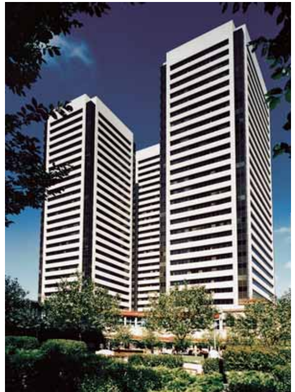
The Sun Life Plaza office towers in Calgary are the site of the first Armstrong ceiling recycling project in Canada. Nearly 250,000 square feet of old tiles were reclaimed.
