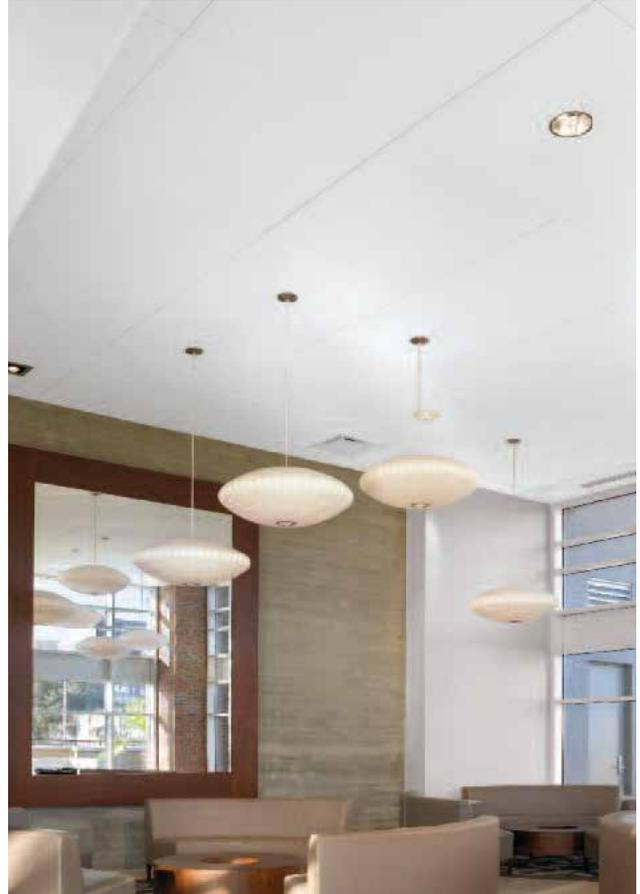
However, even a conventional acoustical ceiling can provide a limited degree of fire resistance. That’s because most fires start small, and may be controlled early by the sprinkler system. A conventional ceiling may thus remain intact and provide resistance to the movement of smoke, fire gases, and spread of flame into the space above.
