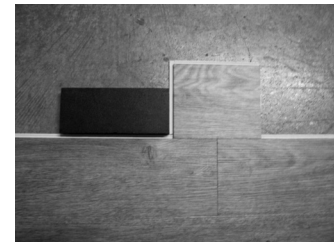
Fig. 7 – Tap side of plank with tapping block.
