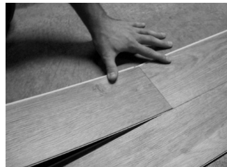
Fig. 5 – Angle end of next plank.
